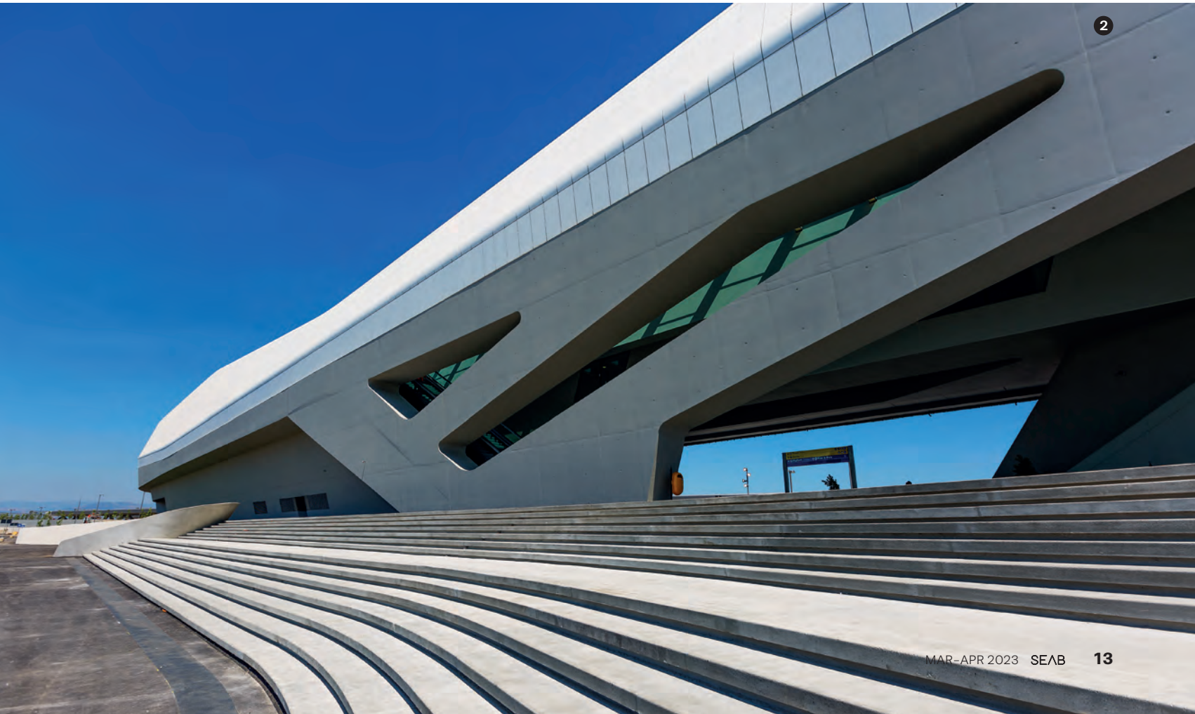
Photos 1 & 2: The surfaces were skimmed with PLANITOP FINE FINISH, which was specifically developed for this site. They were then finished off with MALECH primer and COLORITE BETON paint in a tailor-made RAL colour.
