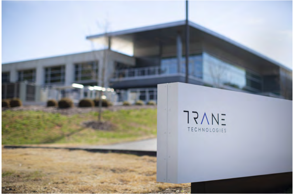
Photo credit: Trane Technologies
