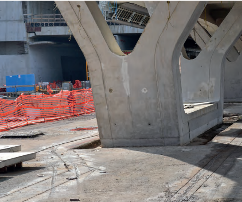
Where required, the concrete was repaired and levelled off with MAPEGROUT T60 and MAPEGROUT LM2K. EPORIP was recommended to seal any cracks in the concrete.
