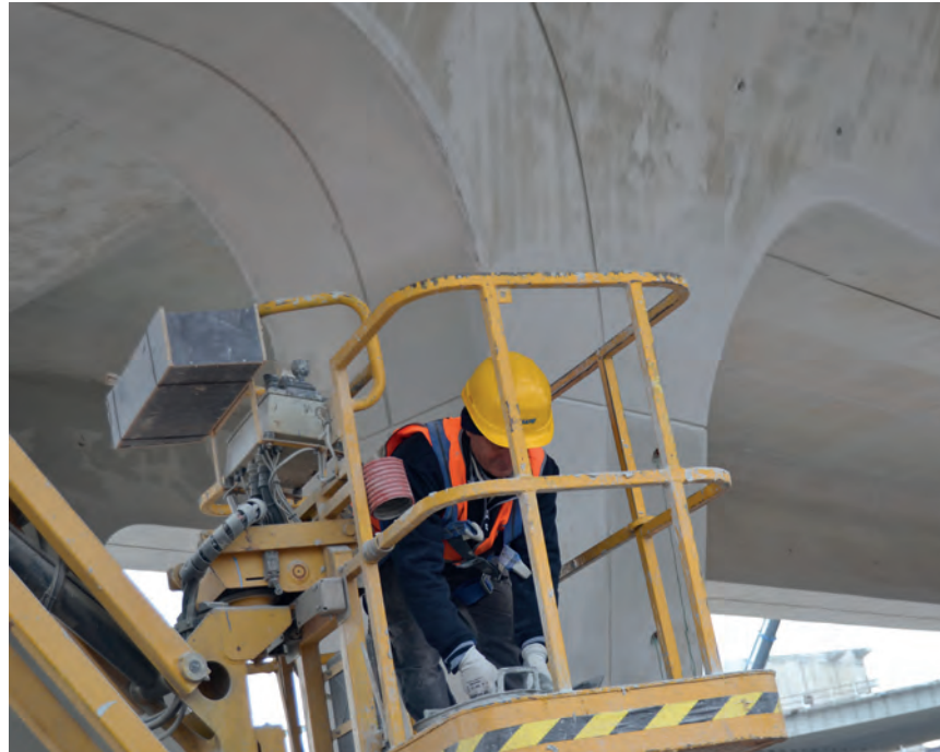
Where required, the concrete was repaired and levelled off with MAPEGROUT T60 and MAPEGROUT LM2K. EPORIP was recommended to seal any cracks in the concrete.
