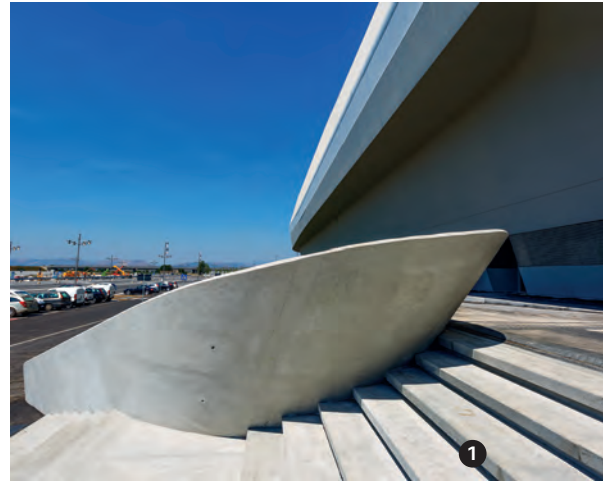
Photos 1 & 2: The surfaces were skimmed with PLANITOP FINE FINISH, which was specifically developed for this site. They were then finished off with MALECH primer and COLORITE BETON paint in a tailor-made RAL colour.
